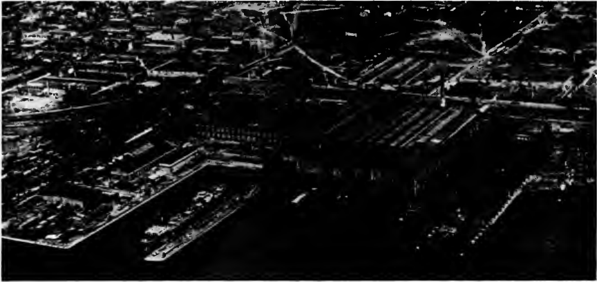
Birdseye view of the plant of the New York Shipbuilding Corporation, showing the three covered ways and the covered fitting out berth. New building ways will be put in along the waterfront to the right of the picture.
